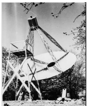
His first using 9 Meter (29ft) was receiving at 3300 MHz, then 900 MHz and finally successful at 160MHz in 1938.
